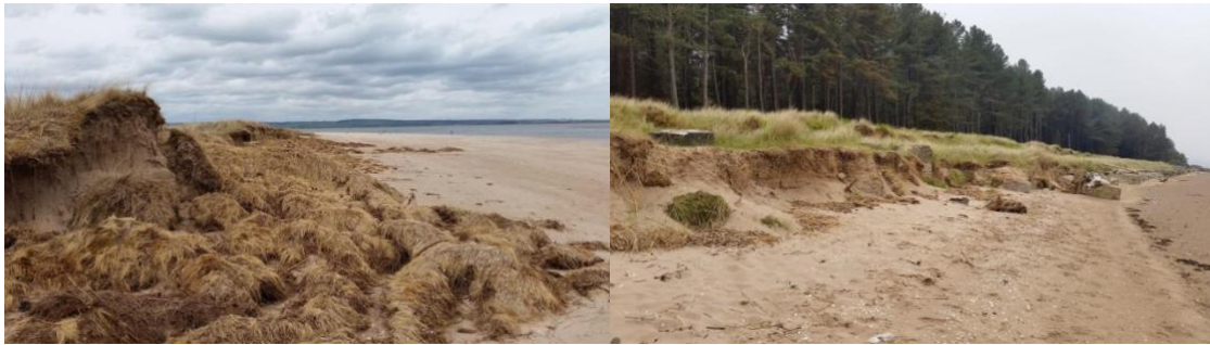
Images of the erosion: Image on the left is in the northeast area and the image on the right is at the north end by the sea fence.
