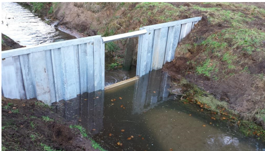
The completed sluice with oak dropboards in place
