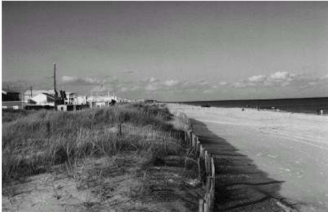
Figure 13. A natural dune system with sand trapping fences: Ship Bottom, New Jersey, USA (Nordstrom, & Mitteager, 2001)
