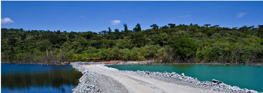
Above: a tailings dam at the Lega Dembi gold mine, Ethiopia
