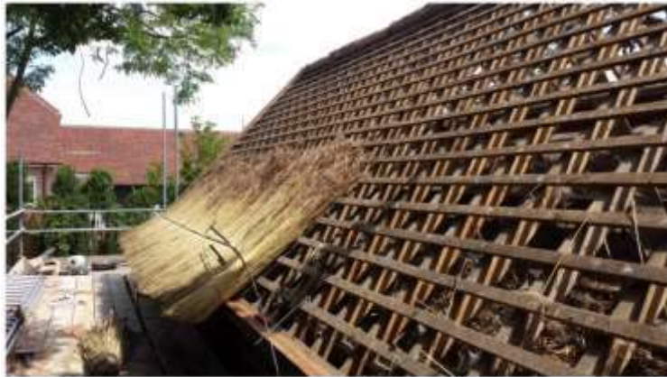
Figure 9 Thatched roofs construction. Source: Danja, 2017 [87]
