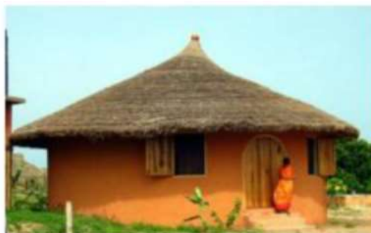
Figure 10 Adobe construction in Ghana. Source: Agyekum, 2020 [80]
