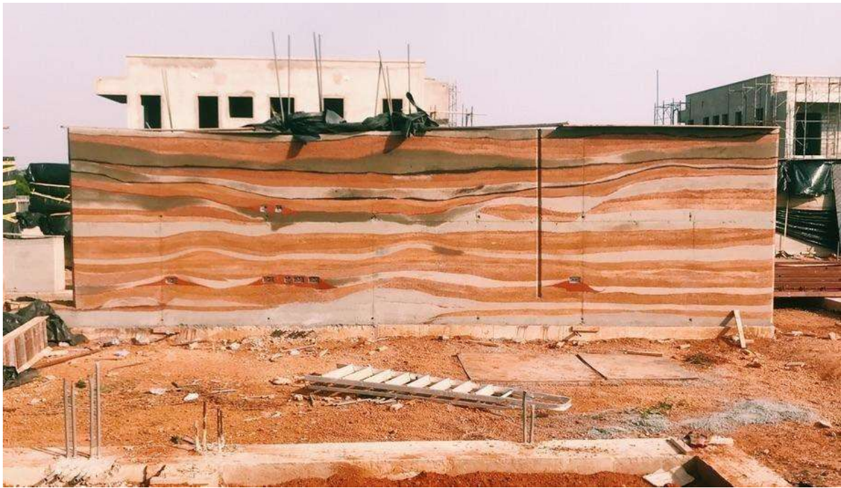
Figure 12 Rammed earth construction in Ghana. Source: Azure magazine (2019) [110]
