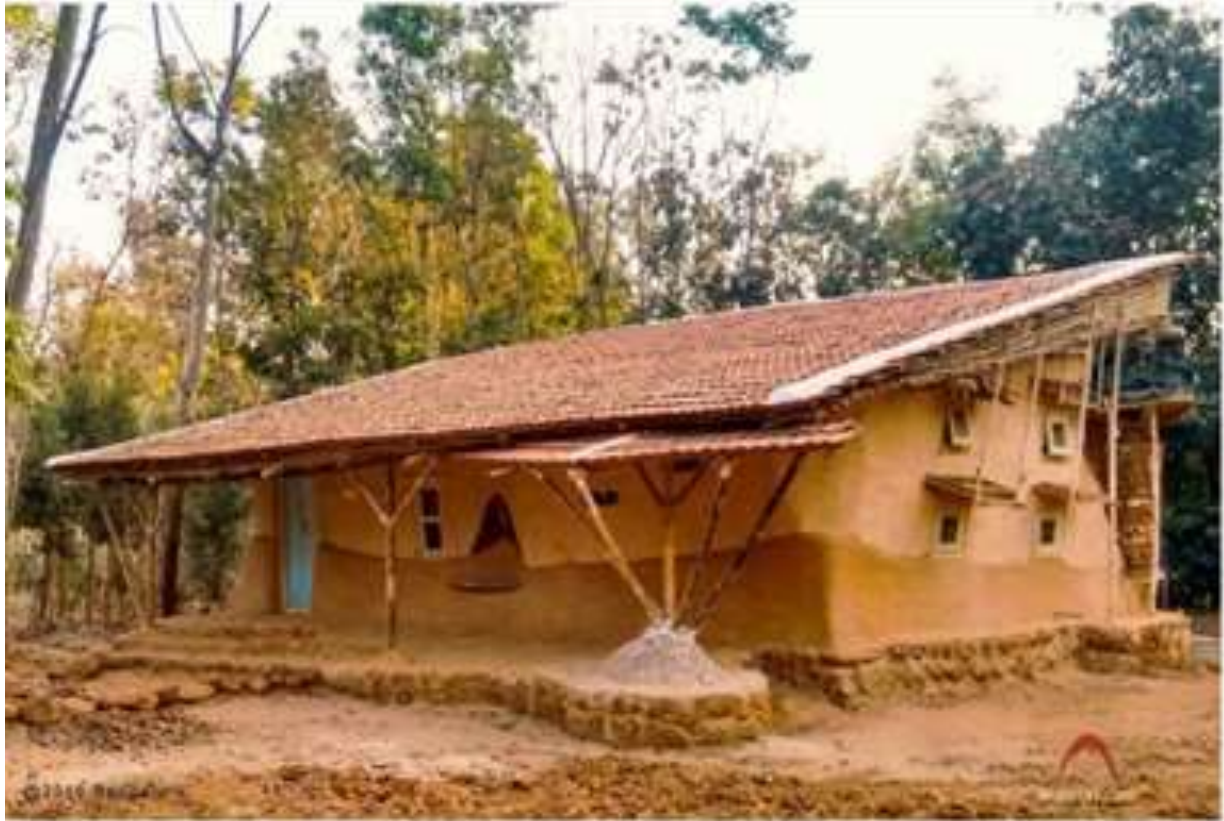
Figure 16 Wattle and Daub construction. Source: Auwalu, 2019 [88]
