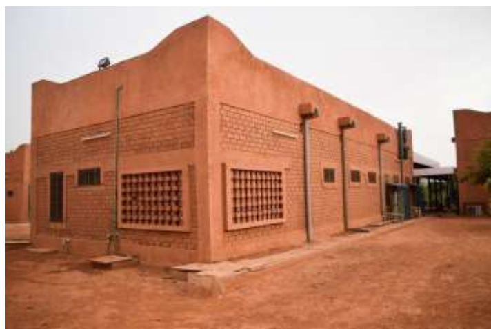
Figure 7 CEB house. Source: Forke, 2017 [69]
