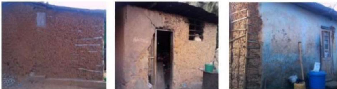
Figure 11: Wattle and Daub in Ghana. Source: Agyekum, 2020 [80]
